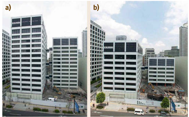
Fig. 57.31a,b Systemic and automated floor-by-floor building deconstruction, Kajima, DARUMA System, Japan (a) early deconstruction phase; (b) later deconstruction phase
