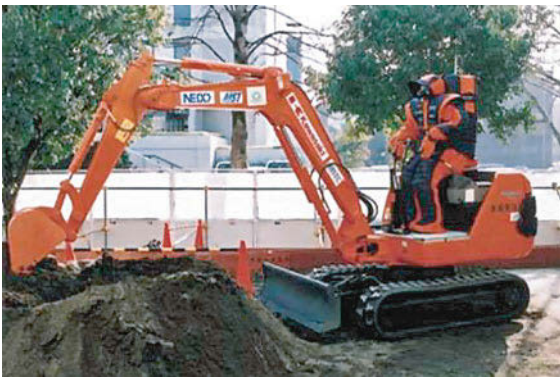
Fig. 67.1 The humanoid robot HRP-1S (HRP: humanoid robot project) driving a backhoe (courtesy Kawasaki Heavy Industries, Tokyu Construction and National Institute of Advanced Industrial Science and Technology (Japan) (AIST)). The robot can be teleoperated by a human operator to control the backhoe remotely. The same robot could potentially interface with many different unmodified machines
