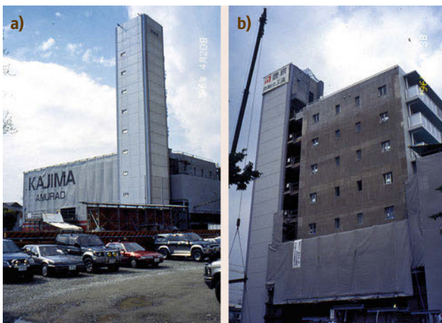
Fig. 57.30a,b The AMURAD Construction Strategy: floor-wise up-pushing of the whole building. Kajima, Japan (a) early construction phase; (b) later construction phase
