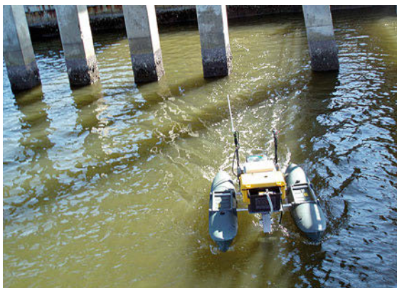
Fig. 60.2 Unmanned surface vehicle exploring the bridge to Marco Island, Florida (courtesy of CRASAR)
