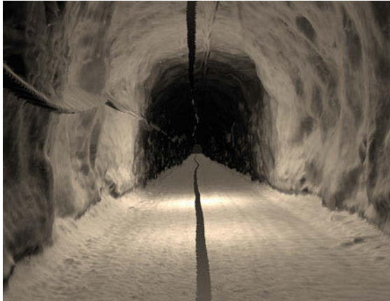
Fig. 59.19 3-D SLAM-generated map of a decline at the Northparkes mine (after [59.112]); the gaps on the floor and ceiling are due to the blindspot between two vertically oriented SICK laser rangefinders; electrical cables can be seen along the left side wall (courtesy of So Jung Yun, 2012)
